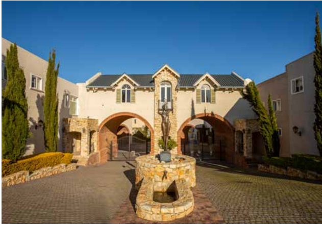
VILLAGE WALK Completed
